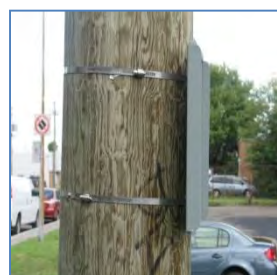
Figure 16, Profile view of pole bracket
